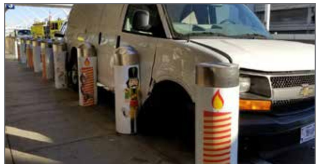
Bollards prevented the van from entering the pedestrian area.
