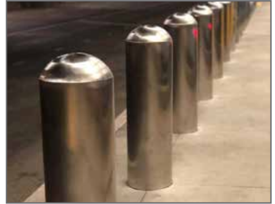
Shallow Mount Bollards at LAX terminals after installation.
